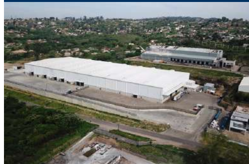
7444m Warehouse For Lease Marianhill, Pinetown
